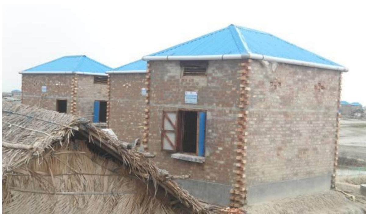
Picture 1: Core Family Shelter Construction in Koyra, Khulna
